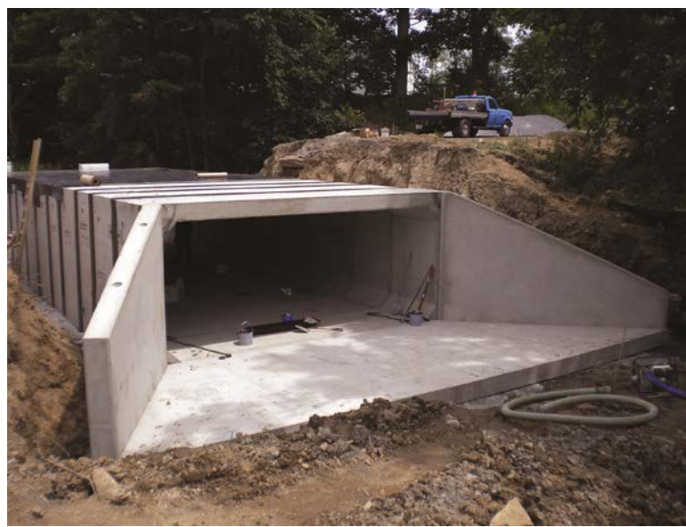
Culvert Replacement
